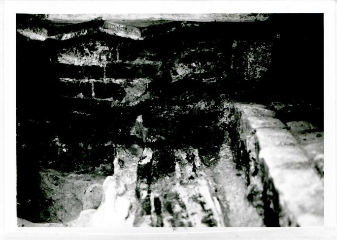
Figure 55a: Eroded support timber at base of column
